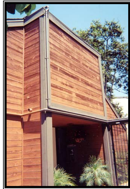
Matching paint can do wonders for camouflaging your pipe run.
